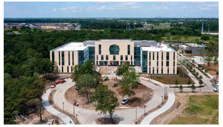
Construction on a new $80 million building to be completed this summer.
